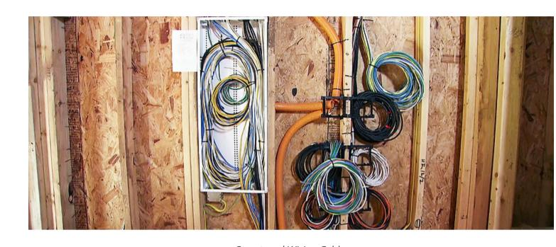
Structured Wiring Cable
